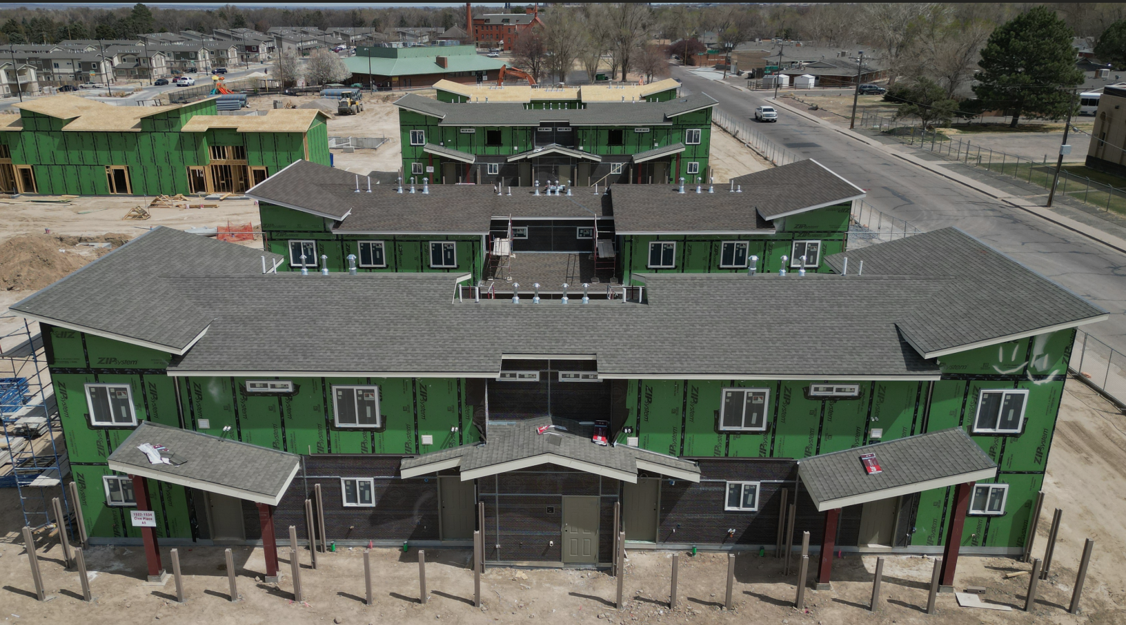
Crawford Townhomes - Under Construction 2023
